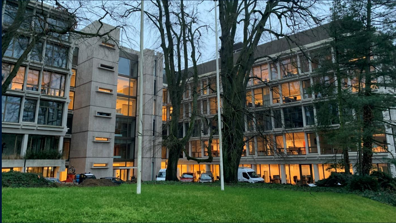
Uccle Townhall. City of Uccle, Archipelago, Socatra (general contractor) + MK Engineering
